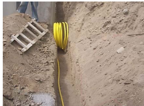
Figure 2. Polyethylene pipe ready to be installed.
