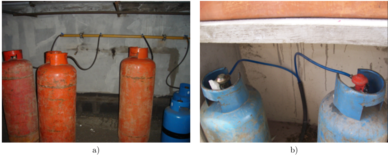
Figura 6. a) Tanks in an area without natural ventilation. b) LPG cylinder with the connecting valve in bad condition.
