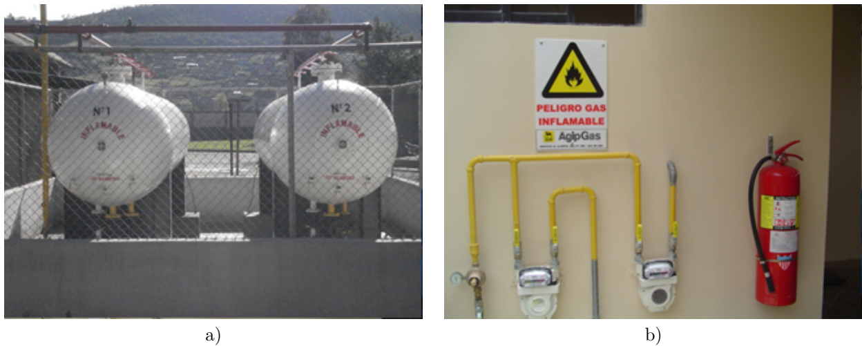
Figura 7. a) Stationary LPG tanks. b) Meters of LPG consumption.
