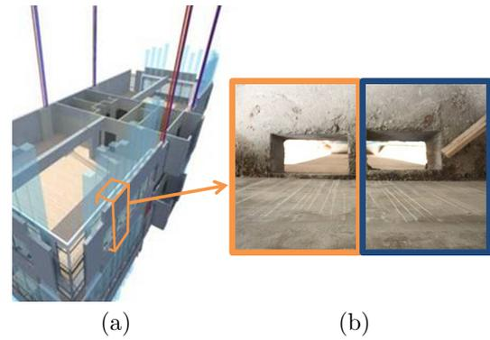
**Figure 2.** a) Portion selected for the simulation. b) Circulation holes made in the slab.
