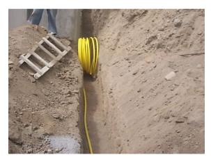
Figure 2. Polyethylene pipe ready to be installed.
